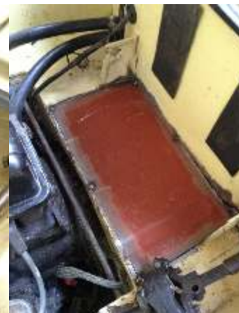
Repair panel tack-welded in place.
